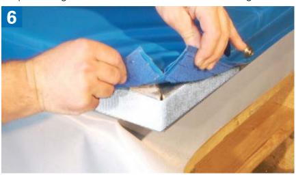
Fix protruding tabs at the corners with the outer edge of the frame (Fig. 6)
