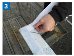
Place the long pad on one corner and apply light pressure to fix it to the frame. (Fig. 4)
